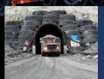
From the surface, the only thing you can see of an underground mine are the two tunnel entrances. The main tunnel is called a decline and the entrance is called a portal. This is used to access the mine. The second tunnel provides ventilation and a fresh air flow throughout the system. The main decline tunnels are around five metres wide and five and a half metres high, just big enough to fit our underground haul trucks and production equipment.
